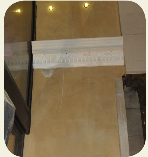
Above: Decorative cove molding has been replicated to include the previously missing crown.
