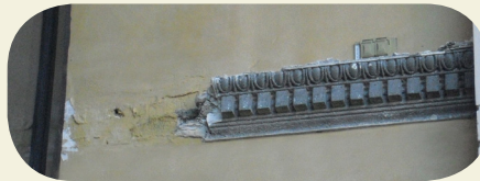
Above: Damaged cove molding shown prior to replication and creation of crown.
